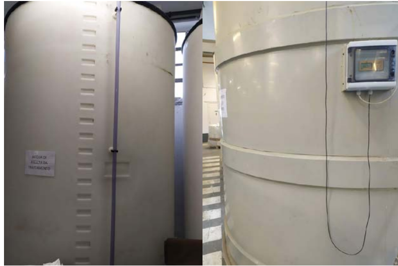
Figure 18. Accumulation and reactor tanks with level indicators of the Gaser treatment plant.
