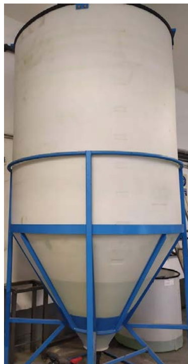
Figure 19. Separation tank with level indicators of the Gaser treatment plant.
